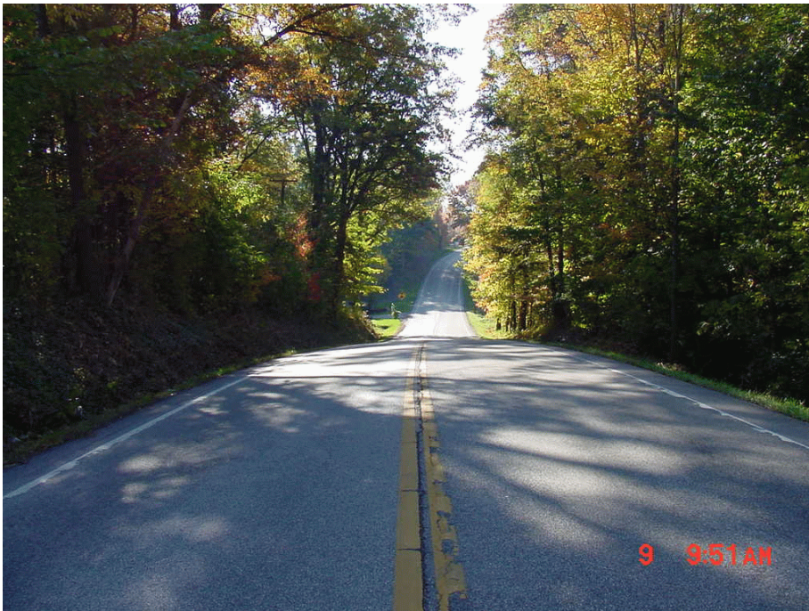
Southbound Approach at 1000 feet- Photo 3
