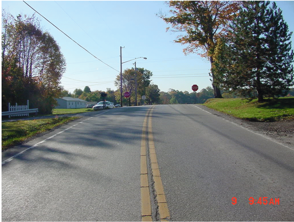
Southbound Approach at 200 feet - Photo 1
