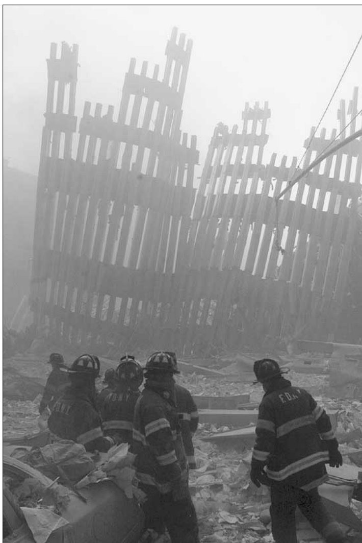
Firemen working near the fallen remains of the landmark 110-story towers.
