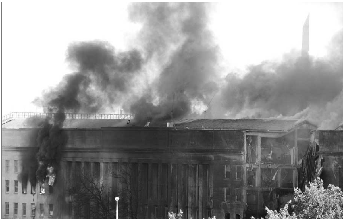
Smoke billowing into the air from the Pentagon following the impact, which caused a portion of one side of the building to collapse.
