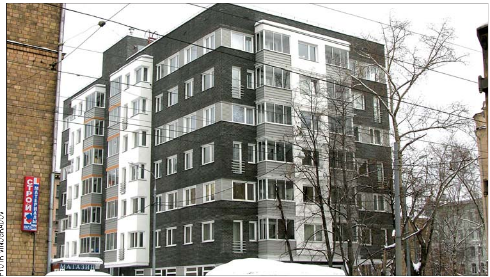
Glazed balconies are a prominent feature of the facade facing Nizhnaya Krasnoselskaya Ulitsa.
