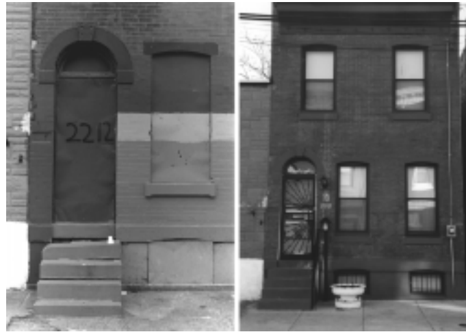
Rehabilitation of a vacant home in North Philadelphia is part of an 18-unit affordable homeownership initiative by Project H.O.M.E. Philadelphia has approximately 30,000 vacant buildings.
