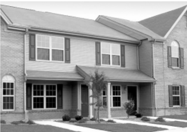
Waggoner Woods, developed by National Church Residences and The Wallick Companies, will provide 175 rental units in the Blacklick area of Franklin County.
