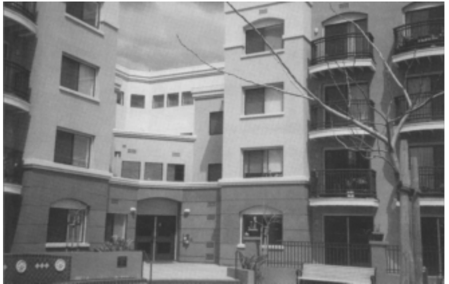
Las Bougainvilleas Senior Housing was developed on 37th Avenue in Oakland by the Spanish Speaking Unity Council. The Unity Council helps build the assets of families and low-income communities through a comprehensive program of sustainable physical, economic and social development. Through its residential and community programs, the Unity Council provides a number of high quality services for more than 250 seniors living throughout the neighborhood.
