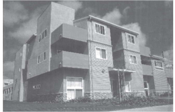
Casa Alegre is a 23 unit building serving homeless people living with HIV in Anaheim. The project provides supportive services to residents including counseling, a food pantry, and health education as well as full access to a built-in entertainment center. Co-developers are Mercy Housing California and the AIDS Services Foundation of Orange County.
