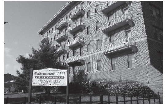
The Housing Production Trust Fund helped purchase, renovate and preserve Fairmont I&II, a 218-unit expiring project-based Section 8 property in the Columbia Heights neighborhood.
