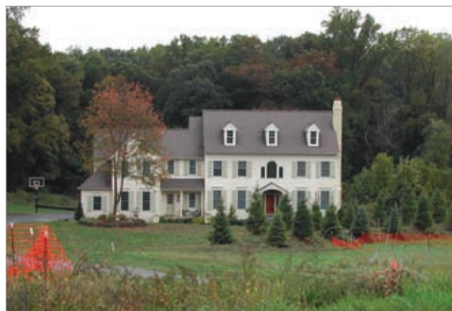
New construction in the woods.
