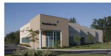
The Fraunhofer USA building, Plymouth, Michigan
