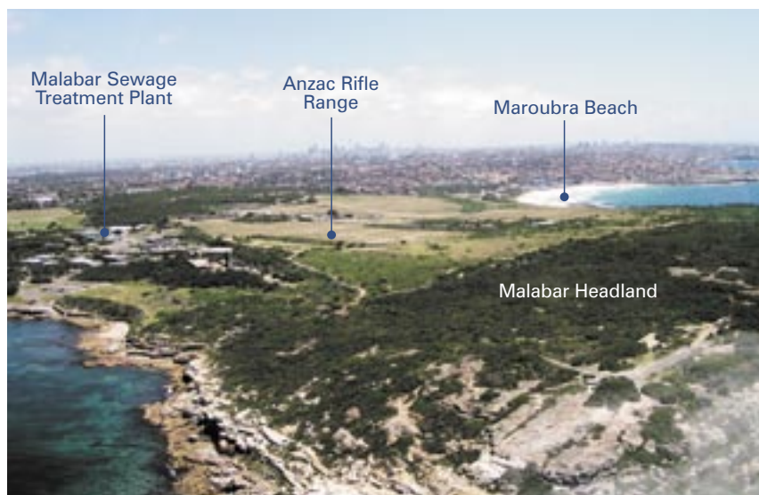
Figure 7.9 Aerial View of 500ML/day Desalination Plant at Malabar
