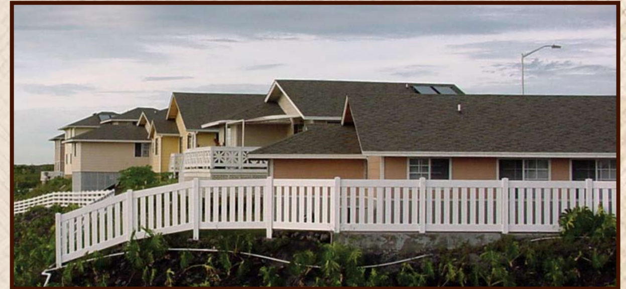
DHHL Home Construction
