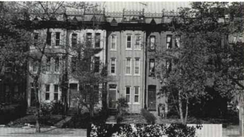
The richness of the Victorian-inspired architecture is exhibited in the decorative pressed bricks and iron cresting of this row at 1816-1826 16th Street (1878).
