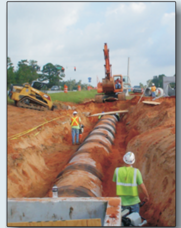
Pictured above: Construction on the Avalon Boulevard stimulus project in Milton.
